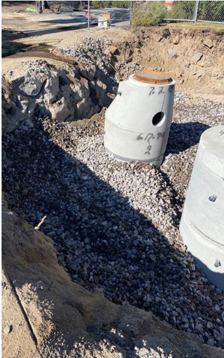
Sedimentation manhole and drywell installation in nearby Desert Woods neighborhood
