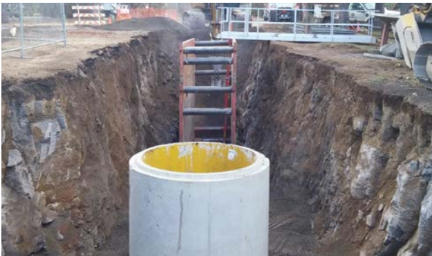
Construction of Southeast Interceptor sewer project
