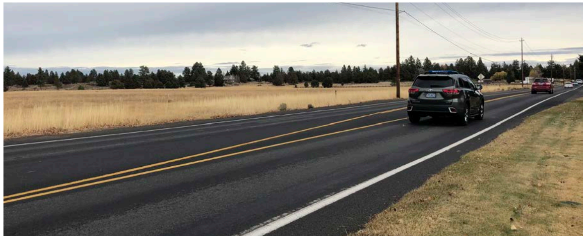
High speeds and narrow shoulders on Knott Road create a high-stress environment for cycling; no sidewalks currently existing on this facility
