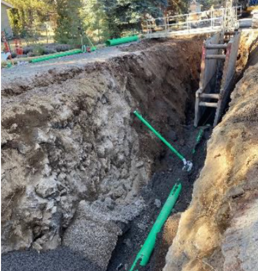
Eight-inch sewer and service lateral
