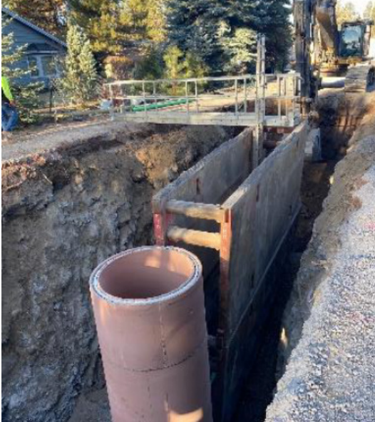
Manhole and pipe install
