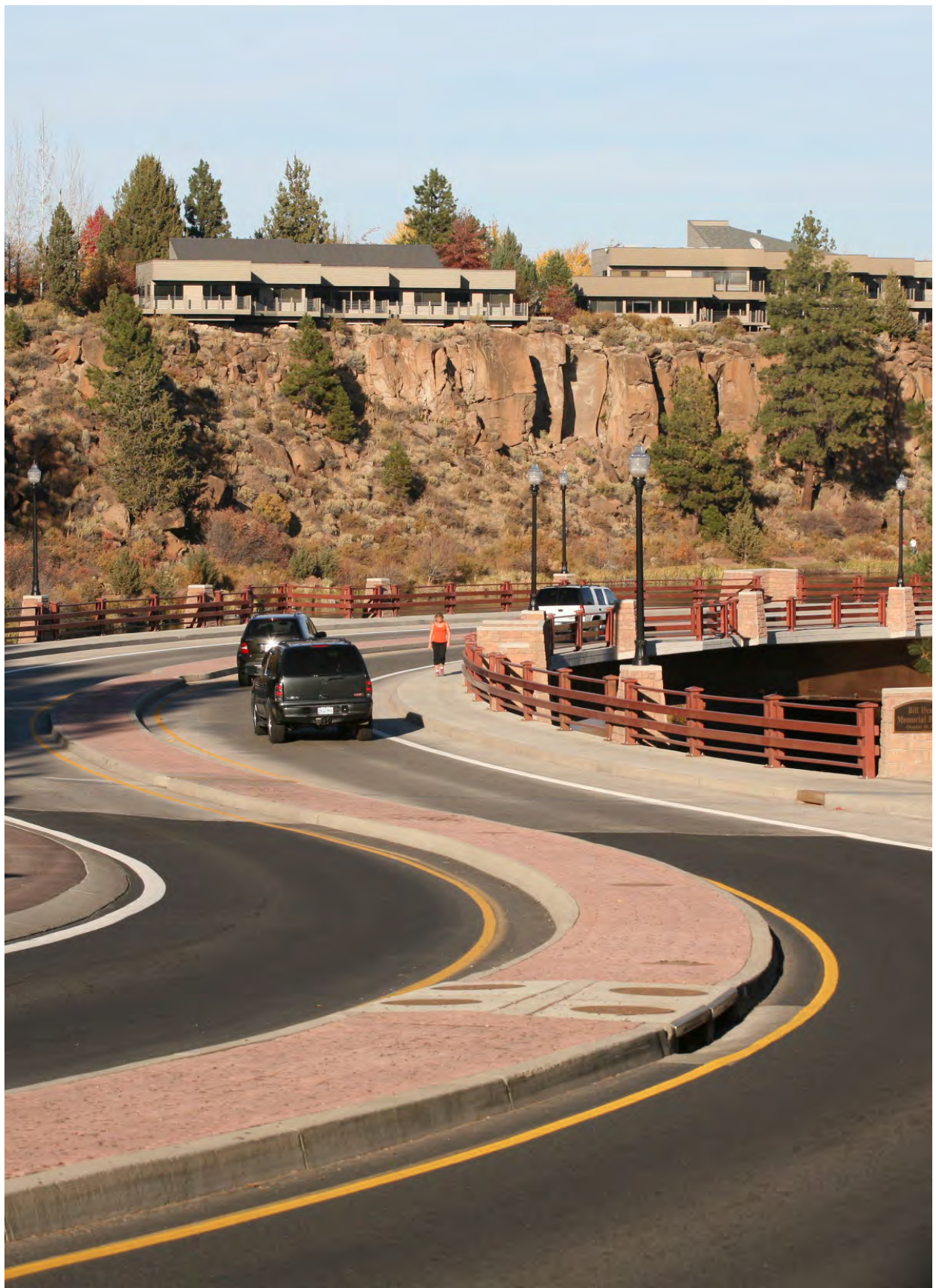
Southern River Crossing
