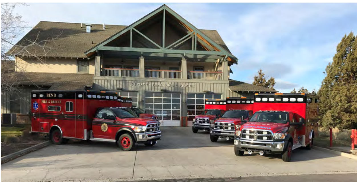
Fire station with emergency services vehicles
